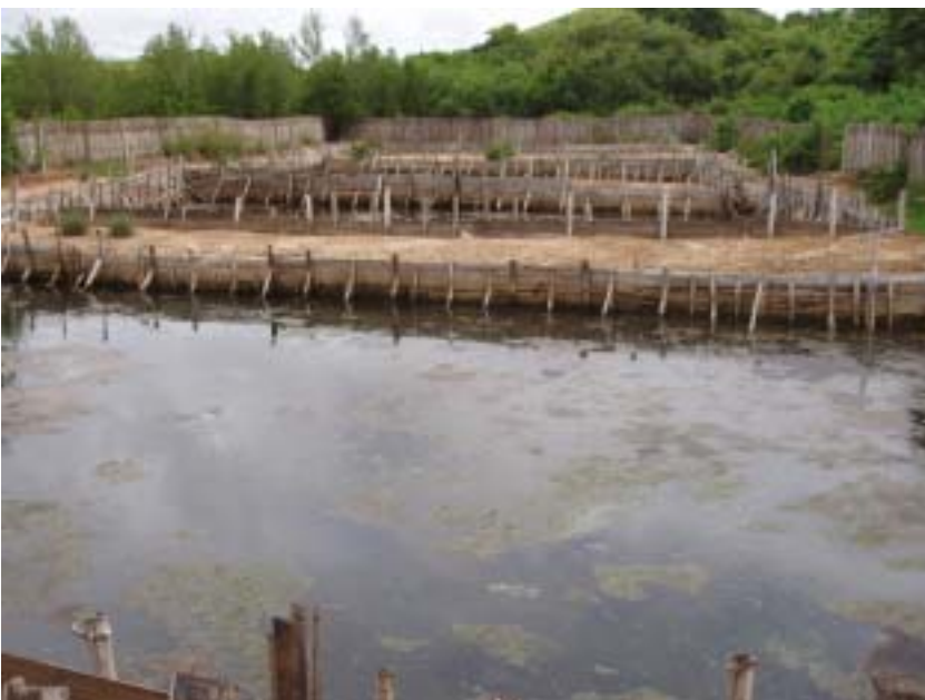
Hatchery facility, waste water treatment ponds
