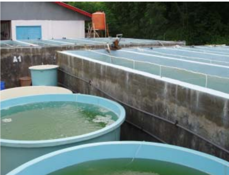
Hatchery facility, algae and rotifer culture units
