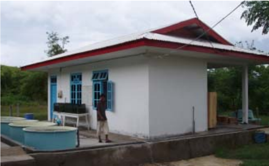
Hatchery facility, laboratory building
