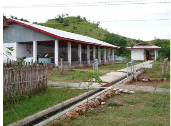
Figure 5. Completed nursery building.
