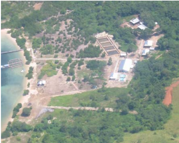
Figure 4. Aerial picture of the hatchery just after completion, March 27, 2003. viewed from the north.
