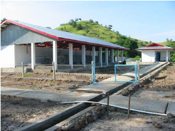
Figure 5. Completed nursery building.
