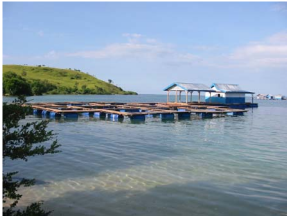
Figure 12. Grow-out unit under construction, to be deployed near a local village (March 25, 2003).
